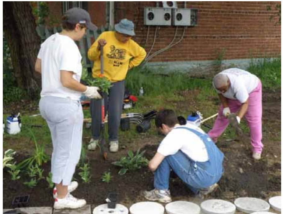
Neighborhood residents building a paved pathway at a community cleanup day. Photo Credit: Liz Colombo
